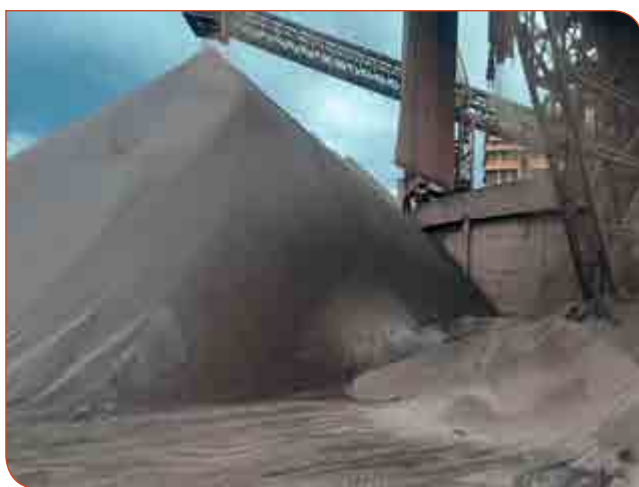
IoBP Division – Pellet Plant
